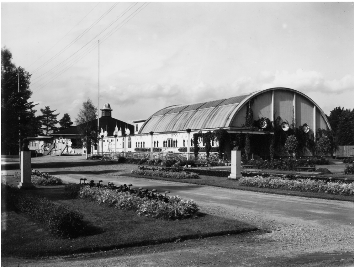
Fig. 13. The People's Park in Sandviken around 1960. By this time many parks, like this one, were professionally landscaped and featured state-of-the-art theaters (middle ground), architecturally-designed restaurants, and improved dance floors (back ground). Photograph by Heed, Länsmuseum Gävleborg (cc by-SA).
